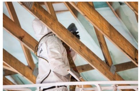
The spray foam system demonstrated excellent adhesion as the roof deck was insulated from the interior.
