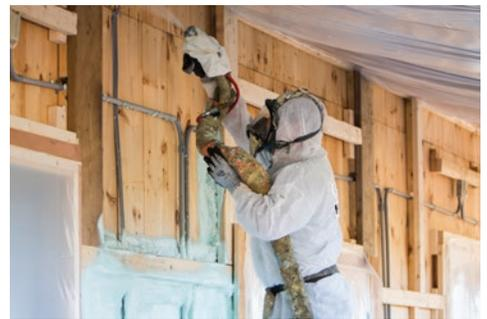
Demilec's new closed-cell spray foam system made with Solstice LBA was sprayed on the building's exterior.
