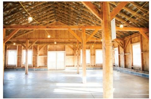
It was important to preserve the historical design of the new structure, including the hand-hewn post and beam construction.
