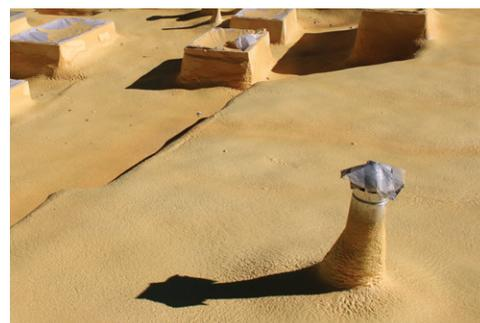
CcSPF is a popular choice given its excellent durability, superior thermal performance and unique ability to contour around the many protrusions and penetrations that must be sealed on complex roofs.
