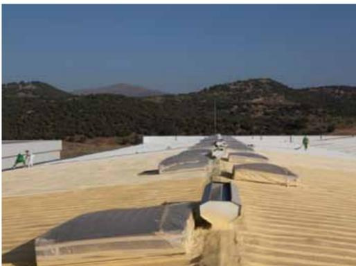
Picture of roofing elements after spraying foam
