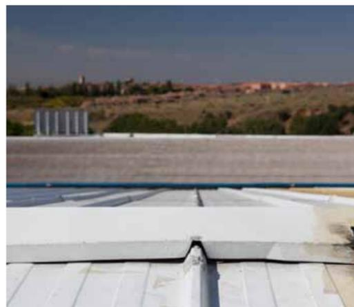
Picture of the condition of the joints before rehabilitation
