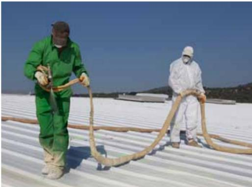
Application of spray foam on roofing
